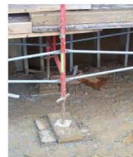
MAXIMUM VERTICAL TIE SPACING WIDER THAN 3'-0" BASES
